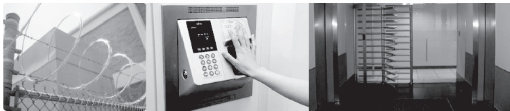
Figure 4.2 Physical security at state-of-the-art data centers includes perimeter security (razor wire), biometric authentication (palm reader), and access control (man trap).
